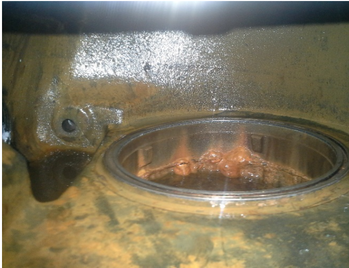
Riser Check Valve Housing Note Corrosion Below Clapper
