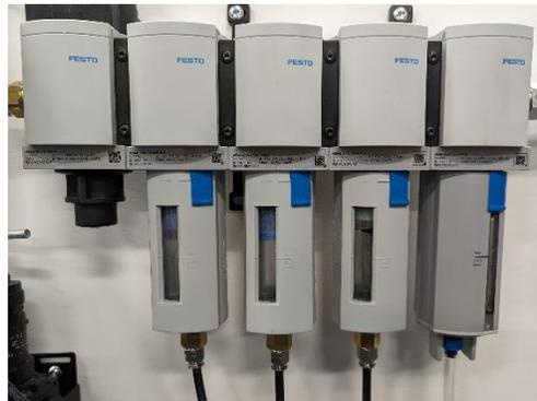
8. Repeat this process for 1-Micron and .01-Micron filters adjacent to water separator, using the kit contents table as a guide to match the filters with the correct housings. Be very careful to do this process **one filter at a time** to ensure the filters do not get mixed in the process.
