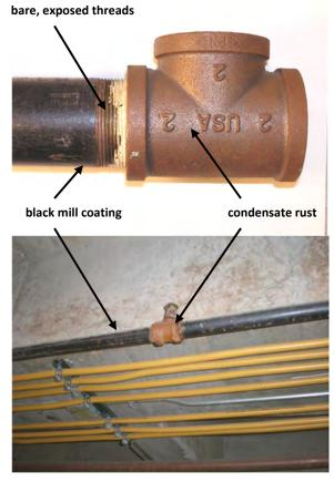
and material cost associated with painting the fire sprinkler system can be quite expensive. In many installations, it is common to leave the installed fire sprinkler system unpainted.
