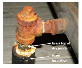
design, the warm moist air can be concentrated at the location above the opened door that introduced the warm air. If enough humid air contacts the pipes they can "sweat" to the point where water drips from them.
