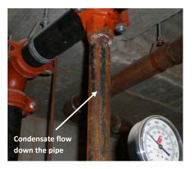
retain the moisture as well. Under conditions where the exterior metal surfaces are moist for extended periods of time, even the galvanized bolts in the couplings can experience corrosion as the zinc layer is dissolved to expose the substrate black steel.
