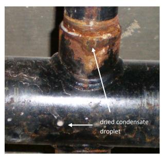
constant use, the amount of pollutant gases in the air at the apex of the building can be considerable. Under some conditions, the localized pH of condensate can fall below 5.0. Condensate at a pH of 5.0 has 1,000 times as much acid in it as municipal drinking water which is typically around pH 8.0.
